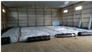
Insul-Tarp was rolled out to cover the leveled floor. Doug mentioned how easy the rolls were to handle...even the 12' x 50' roll!
