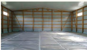
After joining the rolls together with 4" poly tape, it was time to install the wire mesh.
