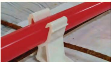
The 1/2" pex tubing used was attached to the wire mesh using ISI's Quip Clips, spaced about three feet apart. The pole barn was ready for concrete.
